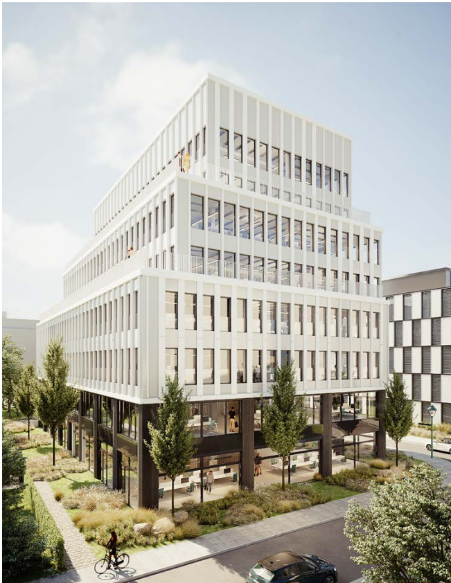
Blick von Südosten / south-eastern view
