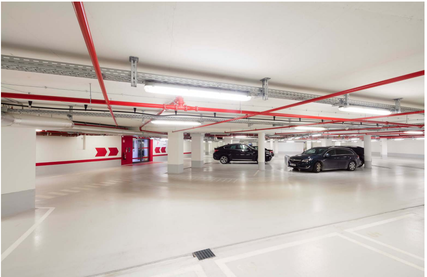
Tiefgarage / underground parking
